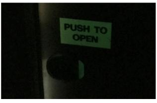
In the event of a power failure, the button to open the door is marked by a luminescent tab, with a luminescent "Push to Open" sign located above it.
